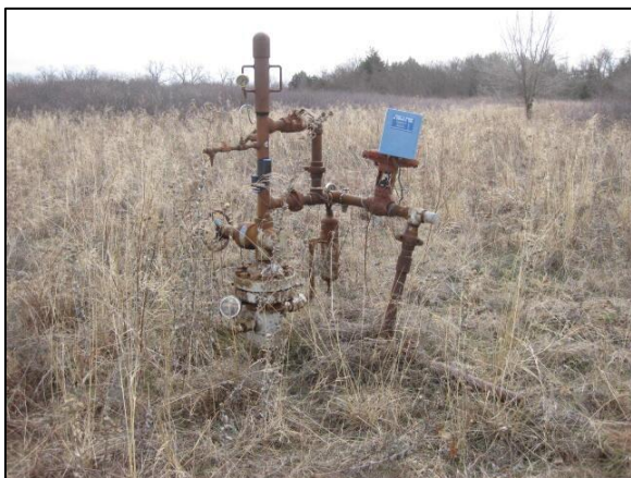
Photo 11: View of well head
