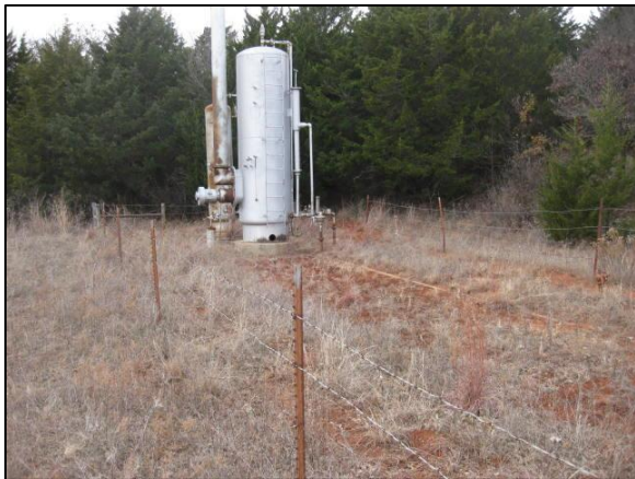
Photo 9: View of the tank battery site
